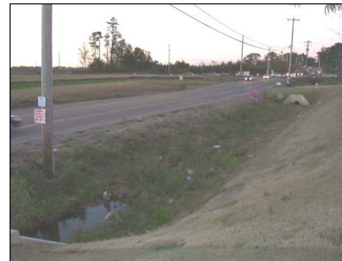
HOUSTON LEVEE: Automotive dominated Houston Levee node shows little consideration for the pedestrian element
